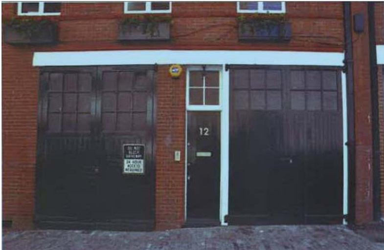
12 Bourdon Street Front Elevation (Door Closed)
